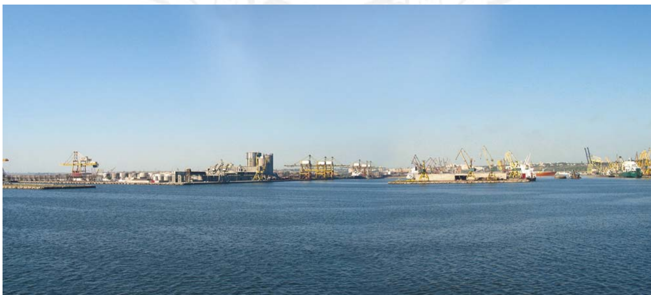
Constanța – Silos at Berth 68 from N & Dock 8, Berth 58 & Dock 9 from E (4.168)
